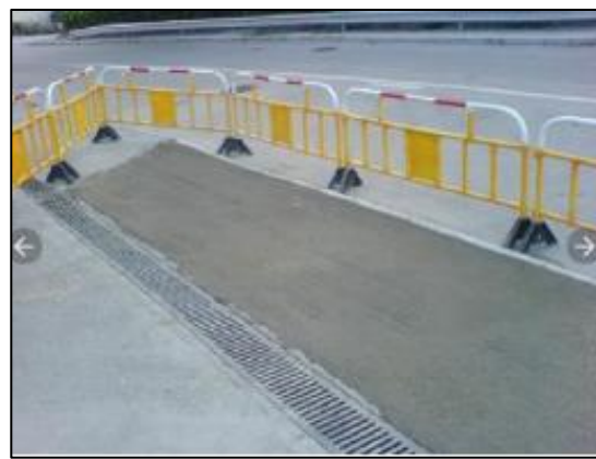
(f) Spare PVC ducts marked on the footway thus C↑D
