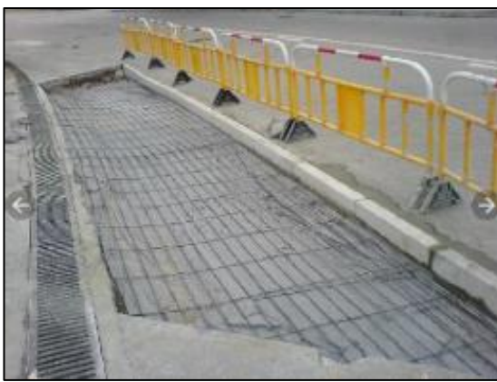
(e) Concrete paving
